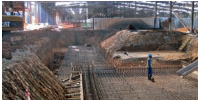
◀ Foundation work in 2016, Piet Retief
