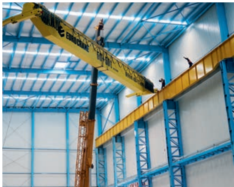
Location expansion in Qingdao: precision work with 2 x 50 metric-ton crane
