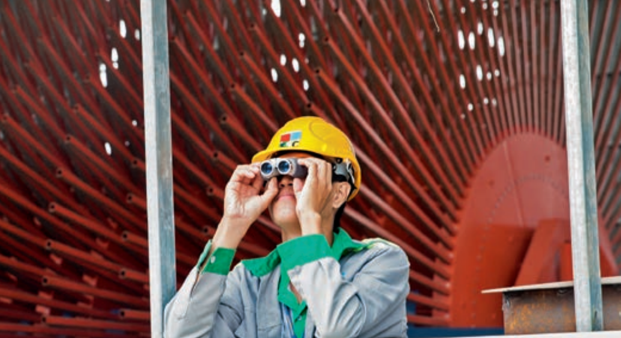
View of cooling tower at FSC Vietnam Corporation
