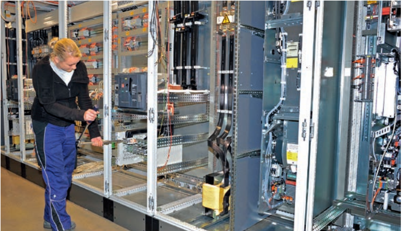
▲ Switch cabinet inspection during assembly
