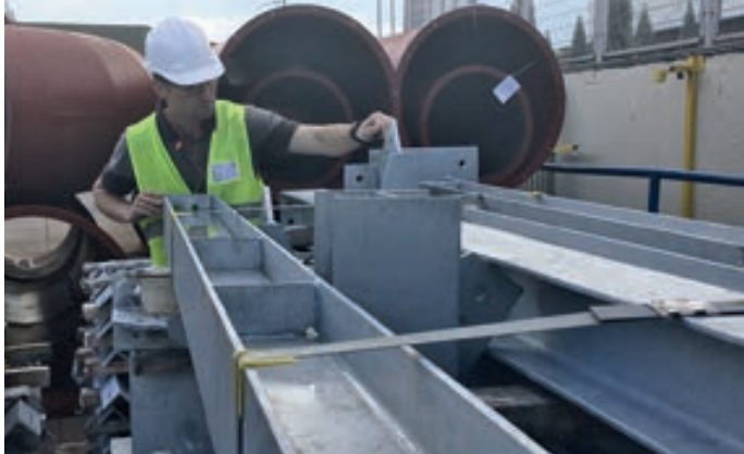
Visual control of galvanized steel components prior to loading
