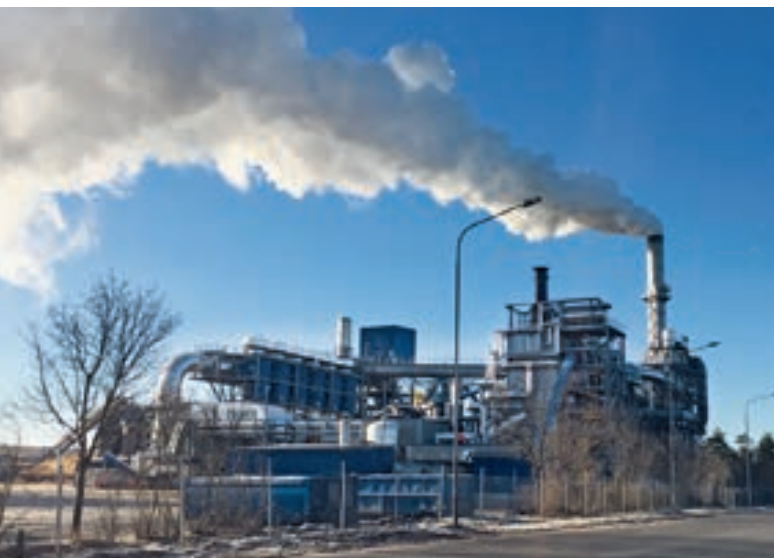
Camsan Entegre, Hendek-Sakarya, Turkey: Büttner fibre dryer and energy plant for the new MDF line
