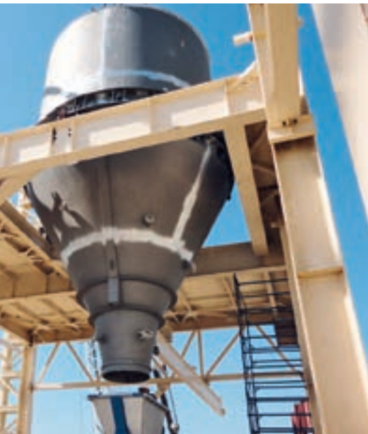
Installation of a chip bin
