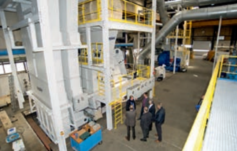
Sifter and piping at Sico's R&D Centre
