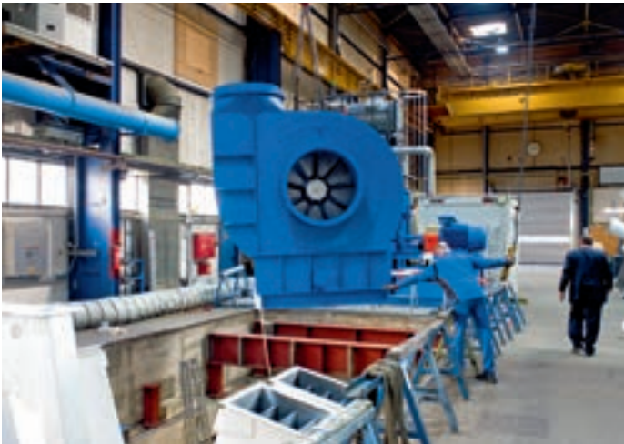
Top left: Lifting the fan, bottom: Heavy-duty tools
