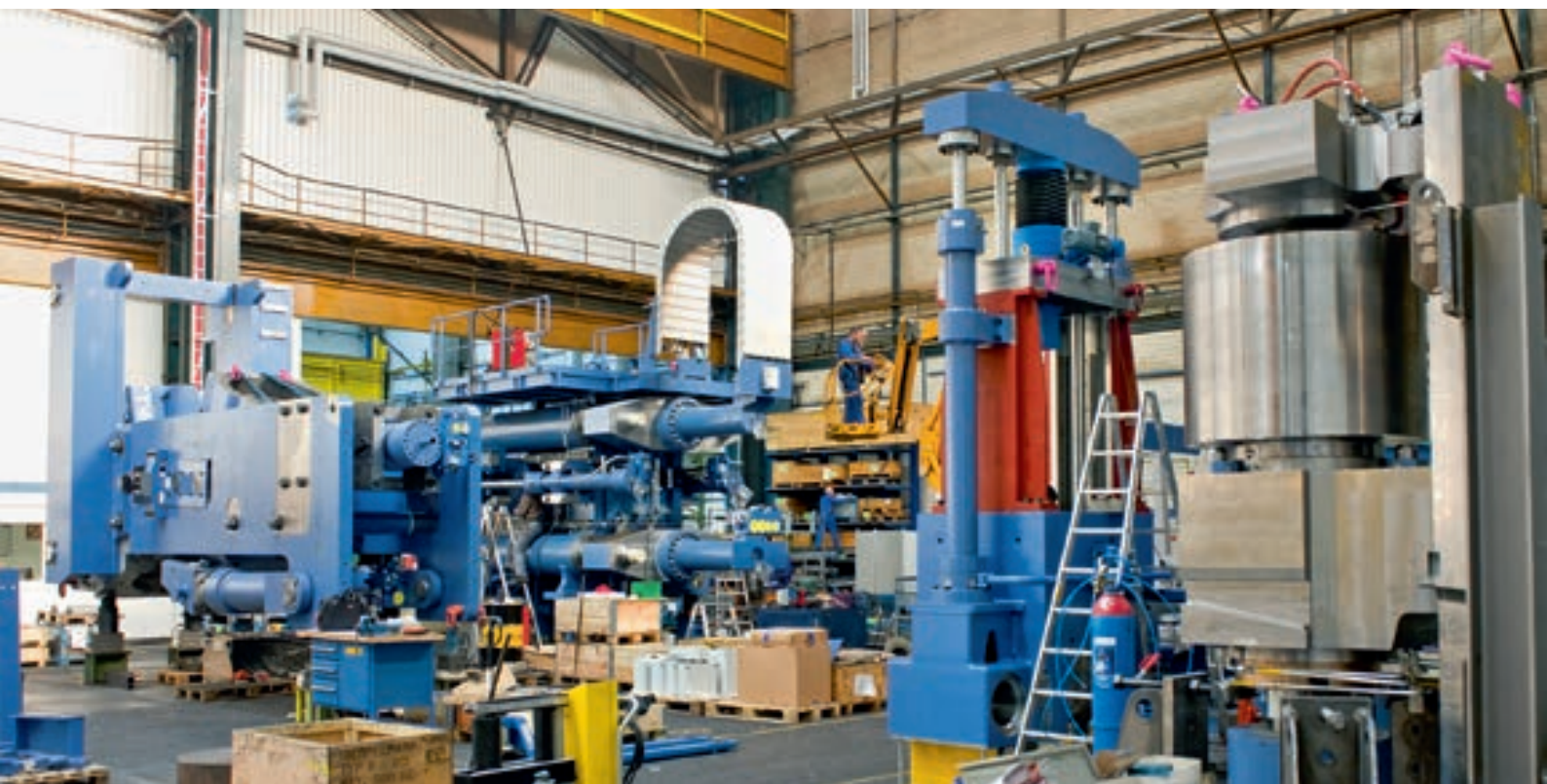
Assembly in Krefeld (from left to right): axial frame, radial frame, upper mandrel bearing incl. mandrel lifter and main rollers
